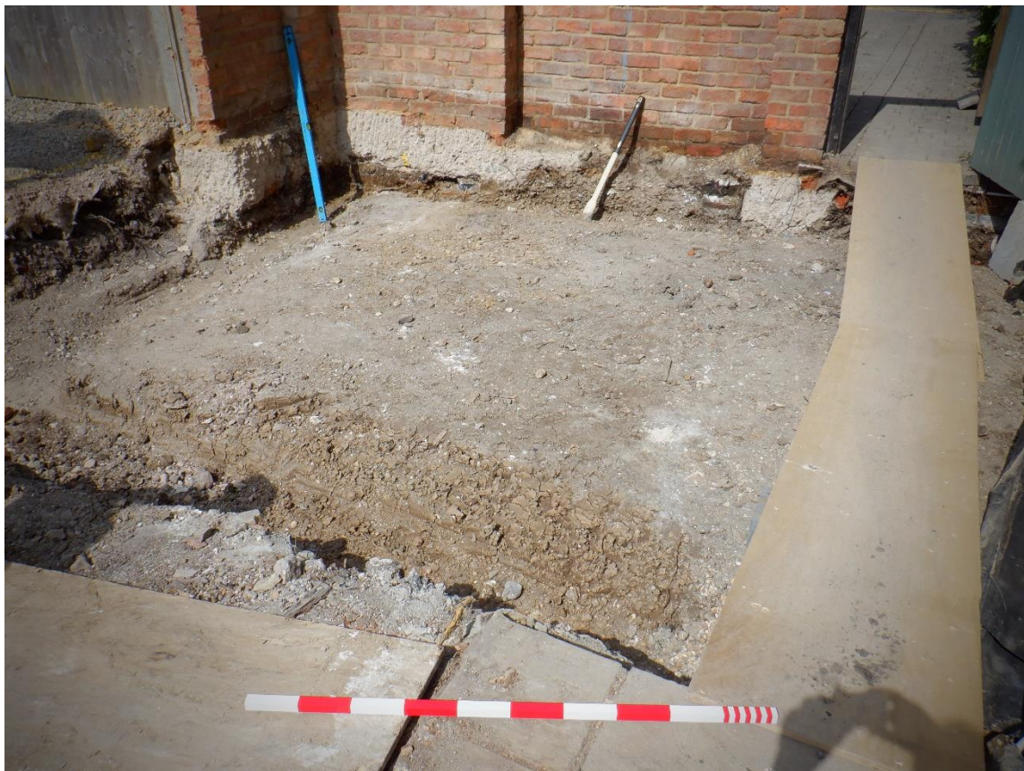
Plate 4. Foundation trenches and slab reduction (looking West)
