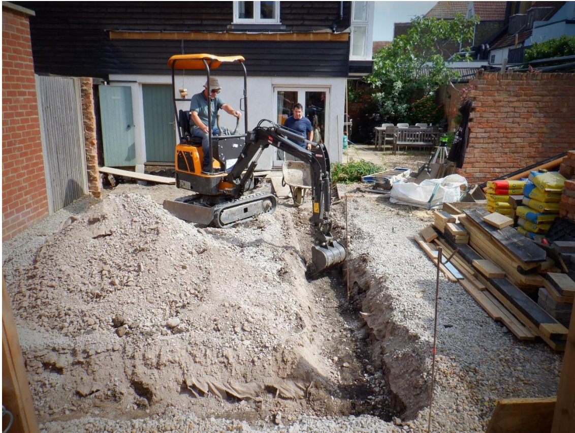
Plate 1. Setting out and starting trenching (looking East)
